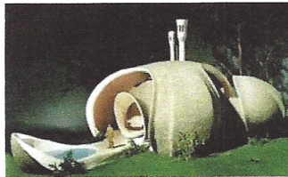
Spray House (1954) Gunite w/o formwork
