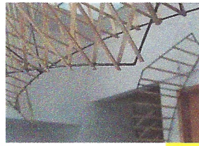
shaped steel bars lath tied with wire
