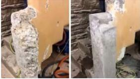
Rounded tops of concrete terrace walls was added only after reinforced walls had set a few days and over the years, the wall caps and surfacing separated from the walls, due to **acid rain seeping in** and **freezing and thawing**. The acid ate into the reinforcing steel cantilevering, causing failure requiring major reconstruction (2001-2002).
