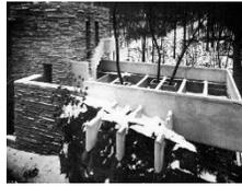
"The **cantilever slabs** here carry **parapets** and the beams. They may be seen clutching big boulders. But next time, I believe, **parapets will carry the floors** - or better still we will know enough to make the two work together as one, as I originally intended."
