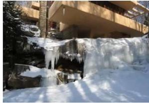
"The roof water is caught by a lead strip built into the concrete above the beginning of the curve. It is not the deluge of water in a storm that hurts any building: it is ooze and drip of dirty water in **thawing and freezing**, increased by slight showers."
